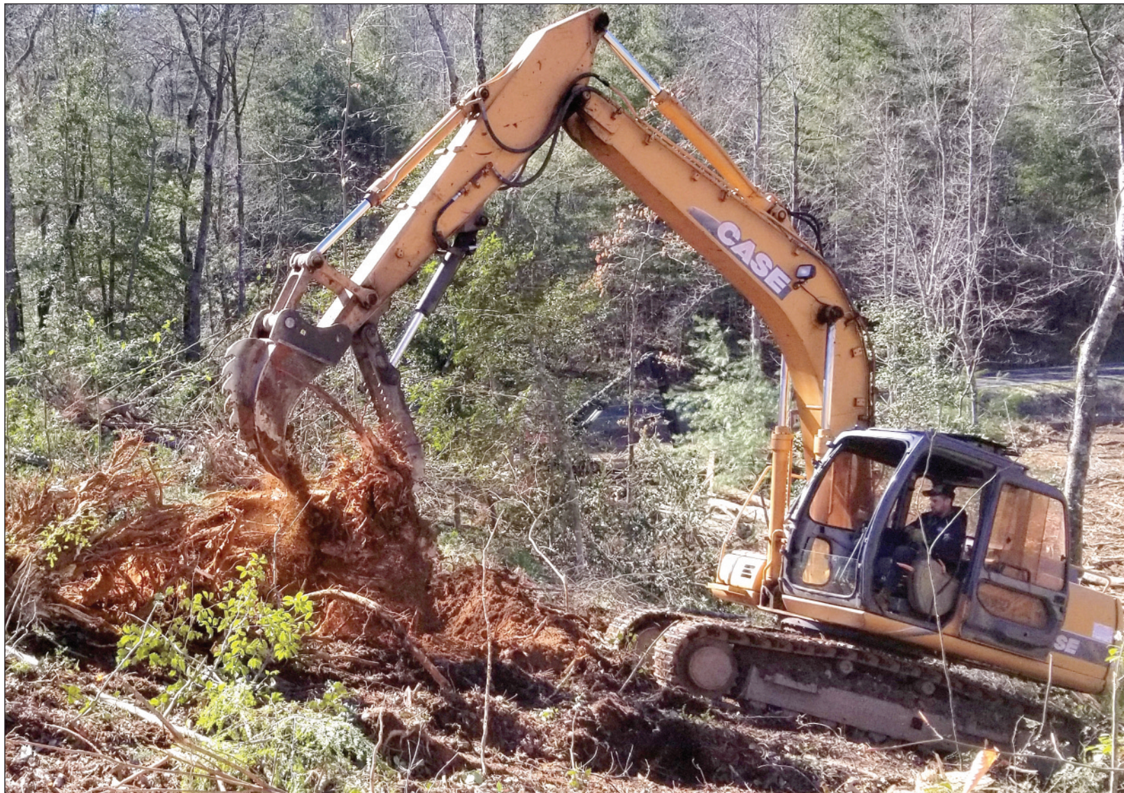
Brian Thompson is not only splitting and harvesting stumps, but also digging trenches for silt fence, loading log trailers and backfilling stump excavations with a Ransome Shark Tooth RST 150 stump splitter/harvester mounted on a Case CX160 hydraulic excavator.
